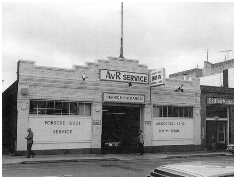
Four early garages, all made of brick, with symmetrical facades. In the top photo are 1) at right, the Alaska Garage, 1349 Larkin Street, by architects Ward and Blohme, 1909-1910; and 2) at left (partially visible), the Graystone Garage, 1335 Larkin, by John H. Powers, 1913-1914 (both extant). In the center photo is the Crown Garage, 1650 Jackson, 1910 (demolished). At bottom is the Pine Garage, 1461 Pine, 1911 (altered).
