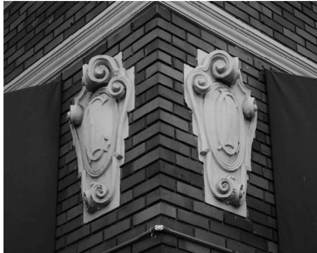
“CL” shield decorations and profiled belt course, Chanslor and Lyon store, 730 Polk Street
