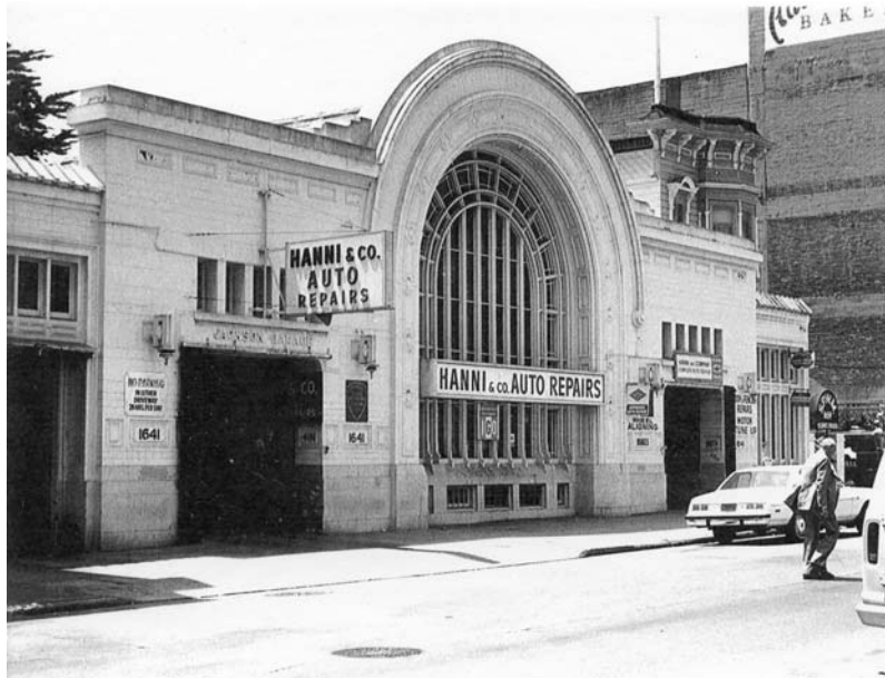
One of the early reinforced concrete garages in the study area: the Jackson Garage, at 1641 Jackson Street, 1914 (extant). Sanborn maps give its capacity as 125 cars. Its architects, the O'Brien Brothers, were the most prolific designers of public garages in San Francisco. This building retains its wood-framed windows, including those in the monumental arch. Photo: Dept. of City Planning Van Ness Avenue Plan, 1980s.
