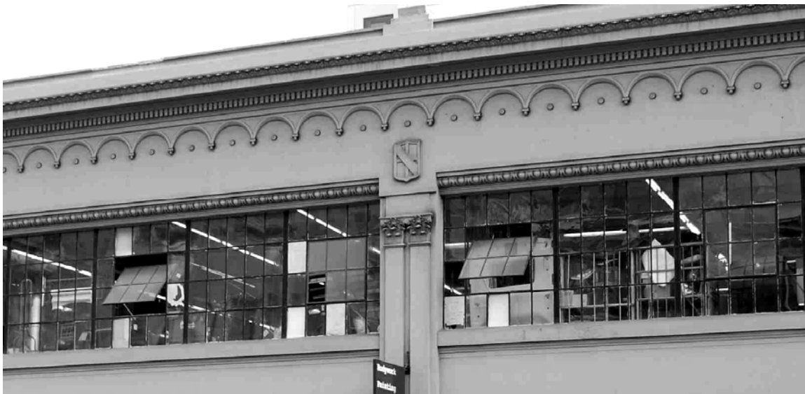
1575-1595 Bush Street (1923), detail of Bush street side, with original industrial steel sash windows
