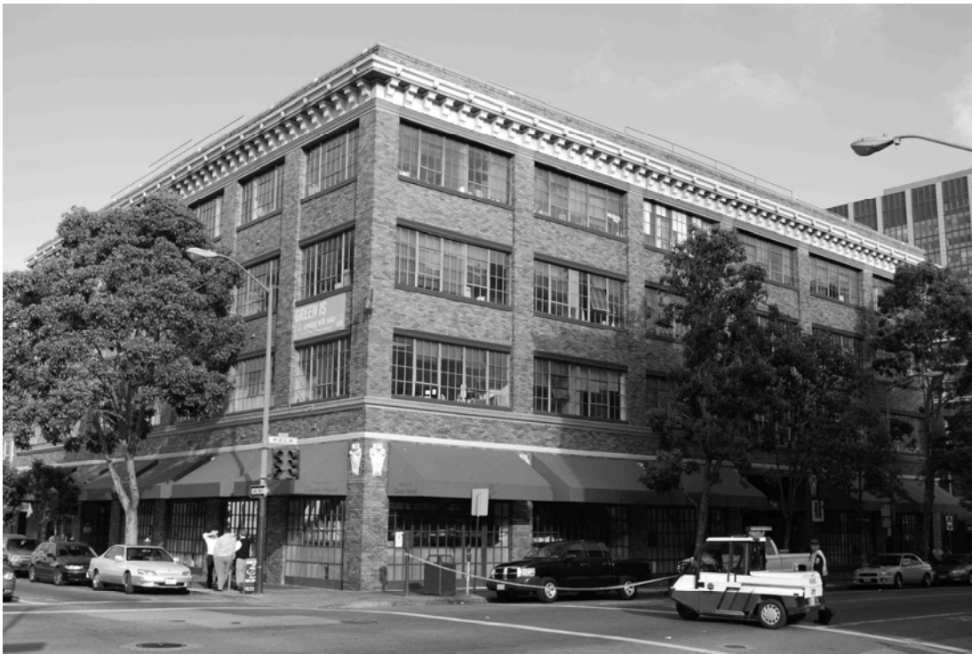
Chanslor and Lyon's wholesale auto parts and supplies store, 730 Polk Street. Built in 1922 to designs by W. L. Schmolle. Integrity is high.
