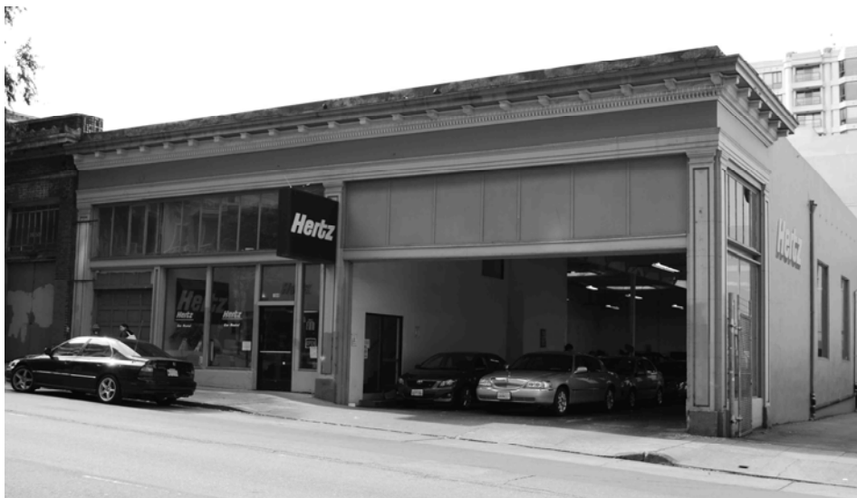
1644 Pine Street, built in 1912-1913 and home to the Michelin Tire Company for six years, to 1919.
