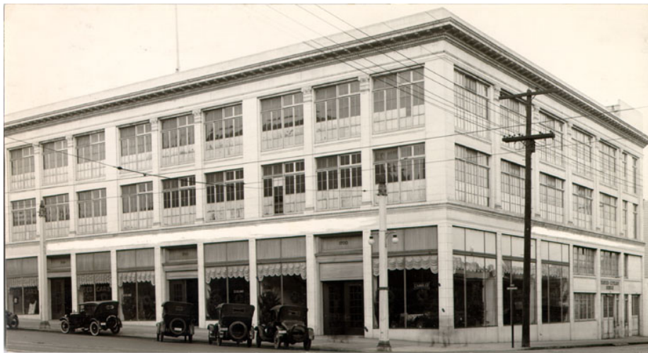
1700 Van Ness Avenue, built in 1919 by MacDonal and Kahn, engineers and contractors, as a showroom for Chandler and Cleveland automobiles. The skeletal construction was lightly decorated with a cornice, profiled belt courses, and classical pilasters. SFPL photo AAD-4652.
