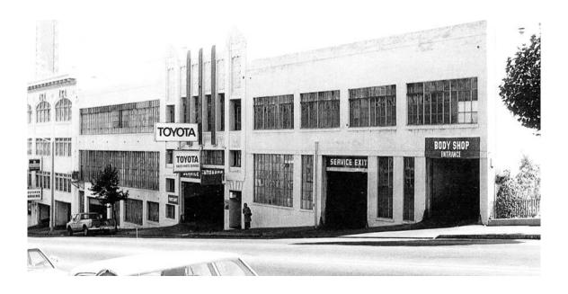
Hanni and Girerd's reinforced concrete auto repair shop, the largest in the study area, at 1765 California Street. The western wing was built first, in 1921, by architect T. Paterson Ross. The ornamental central pavilion and east wing were added in 1927 by Hyman and Appleton. This building's recent conversion to a grocery store retained the original steel sash windows.
