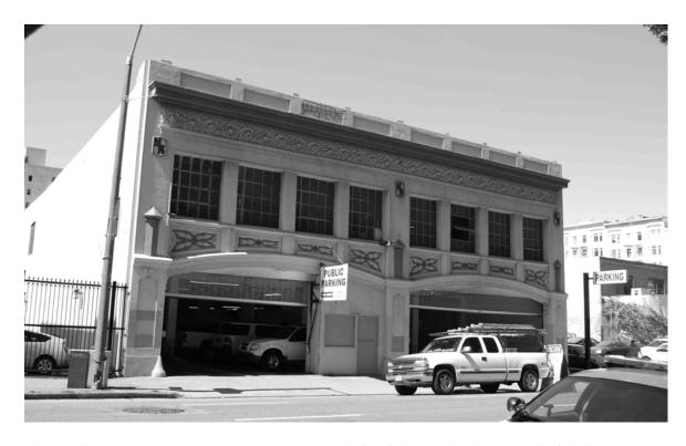
The Admiral Garage, 550 Turk Street. Joseph Pasqualetti, builder, 1924. It is two stories in height, two bays in width, and reinforced concrete in construction. Pasqualetti was a prolific builder of reinforced concrete buildings; here he employed both classical and Gothic decorative details.
