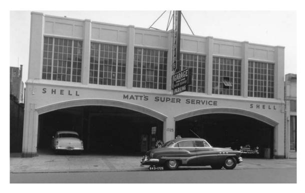
The Marius Bosc Garage, 1725 Sacramento Street, by architect Arthur S. Bugbee, 1923. This symmetrically-designed reinforced concrete garage still stands with all of its industrial steel sash windows intact. Photo: SFPL Assessor's negatives.
