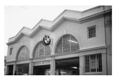
St. Francis Garage, 1240 Post Street, built in 1916 to designs by Sylvain Schnaittacher. Photo by William Kostura, 1983. This was a Class A steel-frame building with a brick front. It had the usual three-bay composition and industrial steel sash windows, but its zig-zag parapet and cornice were unique. This building and the adjacent Heald's College, also by Schnaittacher, were demolished in 1983.
