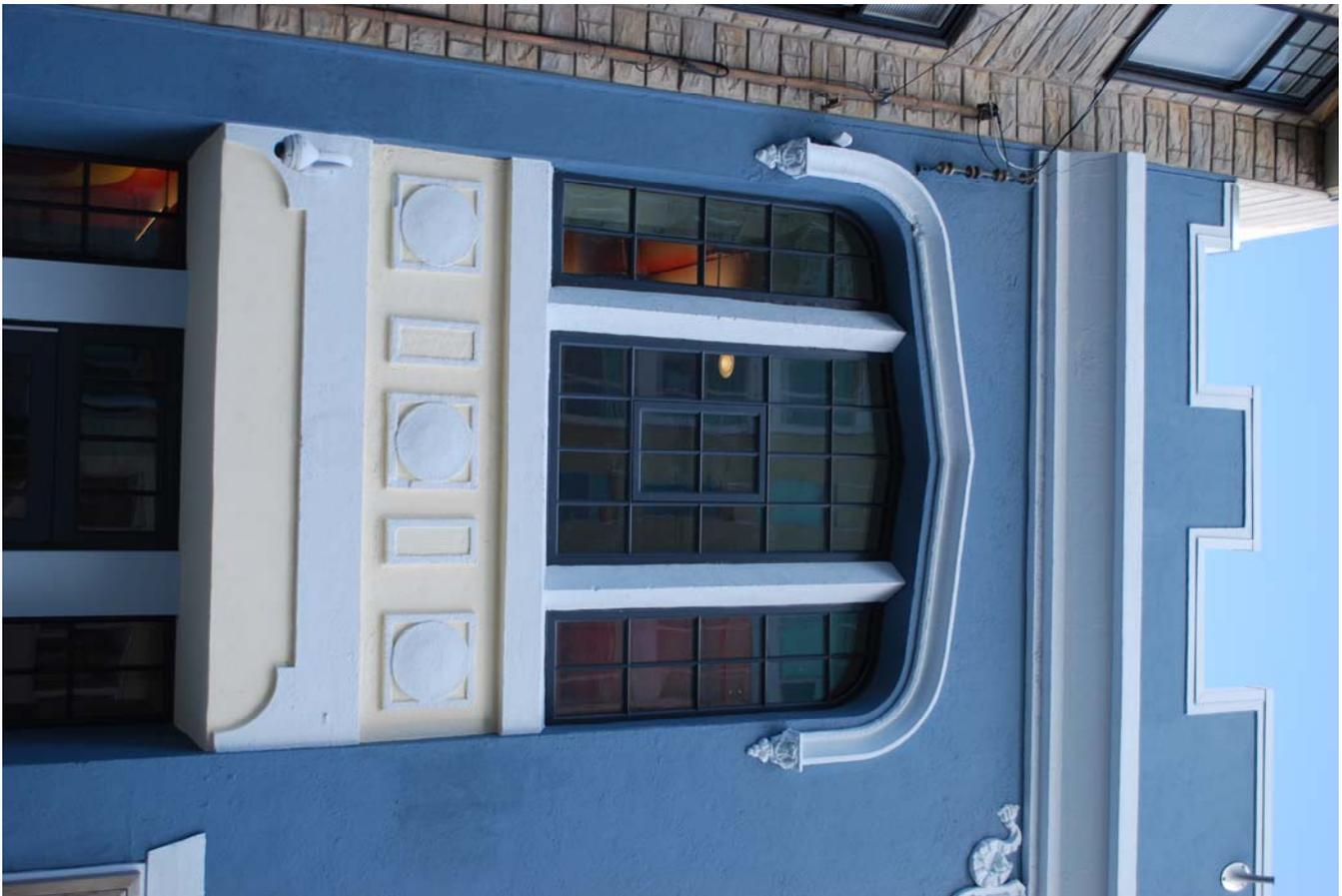
Window and cornice detail, showing new window sash that is virtually identical to the original. The parapet, cornice, drip molding, mullions, paneled spandrel, and lintel over the first story opening (with curved corners) are all original. The treatment of the other two bays is the same. Photo: October 2009.
