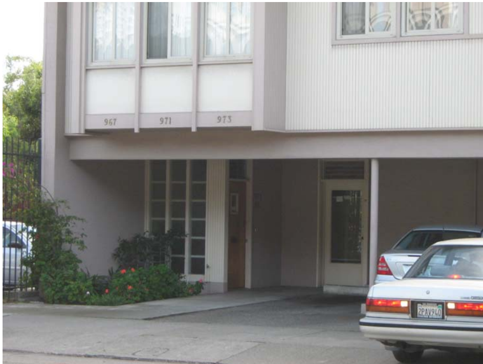
Close up of entrance on Golden Gate Ave.
