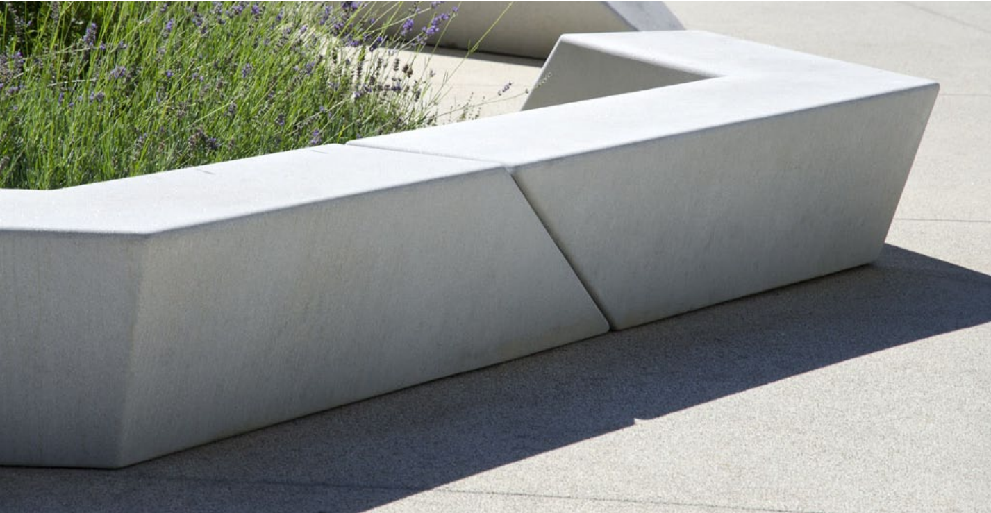
PRECAST CONCRETE UNITS WITH SUBTLE VARIATION IN HUE, SANDBLAST FINISH
