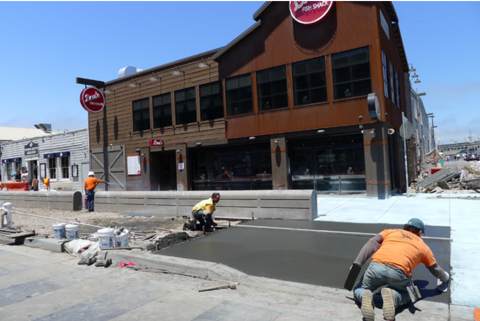
Pavement construction on Jefferson Street between Leavenworth St. and Jones St.
