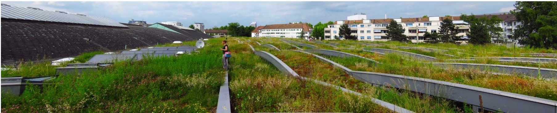
Figure 11 – a $3/sf living roof recently installed in Switzerland, where many years of supportive policy and system simplification have led to significant decreases in first cost
