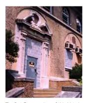
The first floor openings of this historic building have been filled with cinder blocks and the doors, window sash, and frames removed for safe keeping. The security metal door features heavy duty locks. Photo: NPS files.
