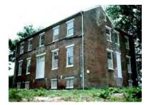
This building has been successfully mothballed for 10 years because the roof and walls were repaired and structurally stabilized, ventilation louvers added, and the property maintained. Photo: NPS files.
