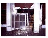
Loose or detached elements should be identified, tagged and stored, preferably on site. Photo: NPS files
