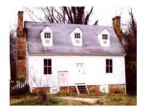
Regrading has protected this masonry foundation wall from excessive damp during its 10-year mothballing. Note the attic and basement vents, temporary stairs, and interpretive sign. Photo: NPS files.
