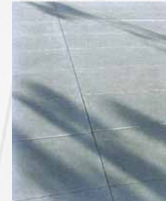
Required saw-cut joints
