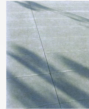
Required saw-cut joints
