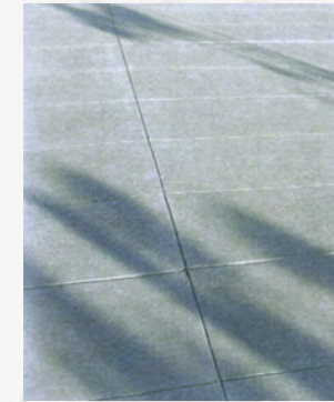
Required saw-cut joints
