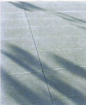
Required saw-cut joints
