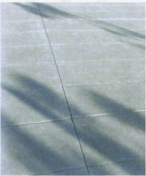
Required saw-cut joints
