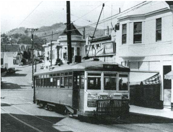
Glen Park's commercial area was built before automobiles began to shape the design of cities. The result is a tight knit walkable and transit-friendly shopping district.
