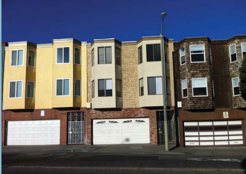
Garages and vehicle entrances disrupt the commercial district's flow of storefronts, introduce conflicts with pedestrians, remove on-street parking spaces, and generally create an uninviting street environment.
