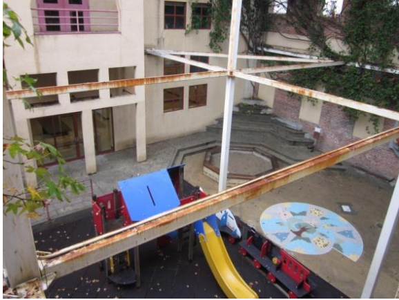
Underused Playground in Uninviting Space
