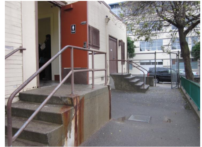
2 Poor ADA access to clubhouse and around park site
