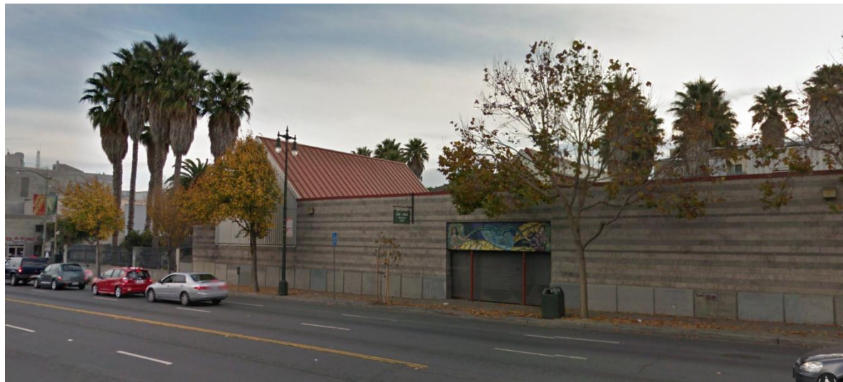
Uninviting Building Entry
