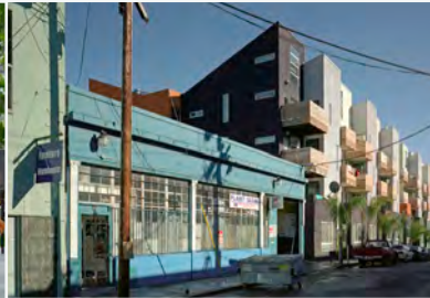
Diversity of Buildings and Architecture
