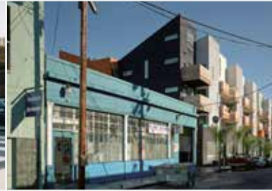
Diversity of Buildings and Architecture
