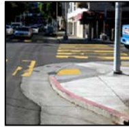
Install corner curb bulb
