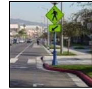
Install mid-block curb bulb
