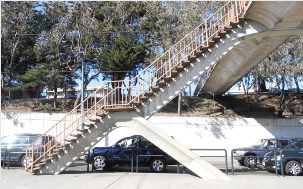
Precast stair treads and steel picket railing at stacked arch columns.
