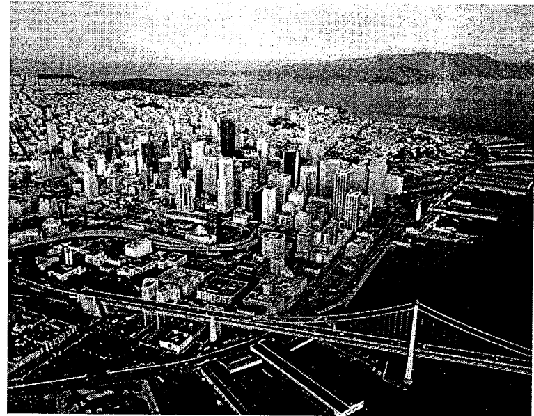
San Francisco Waterfront After the Route 480 Demolition
