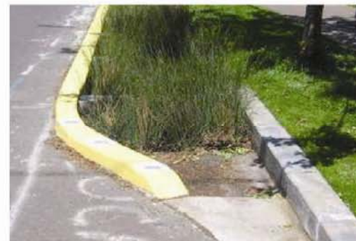
FLOW-THROUGH PLANTER FOR STORMWATER MANAGEMENT
