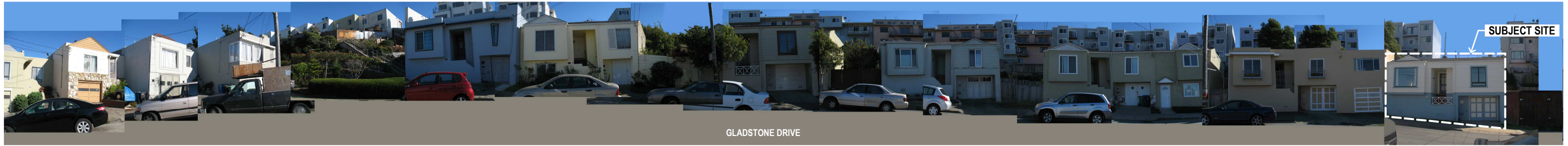
SUBJECT AND ADJACENT BUILDINGS TO THE EAST ON GLADSTONE DRIVE (LOOKING SOUTH)
