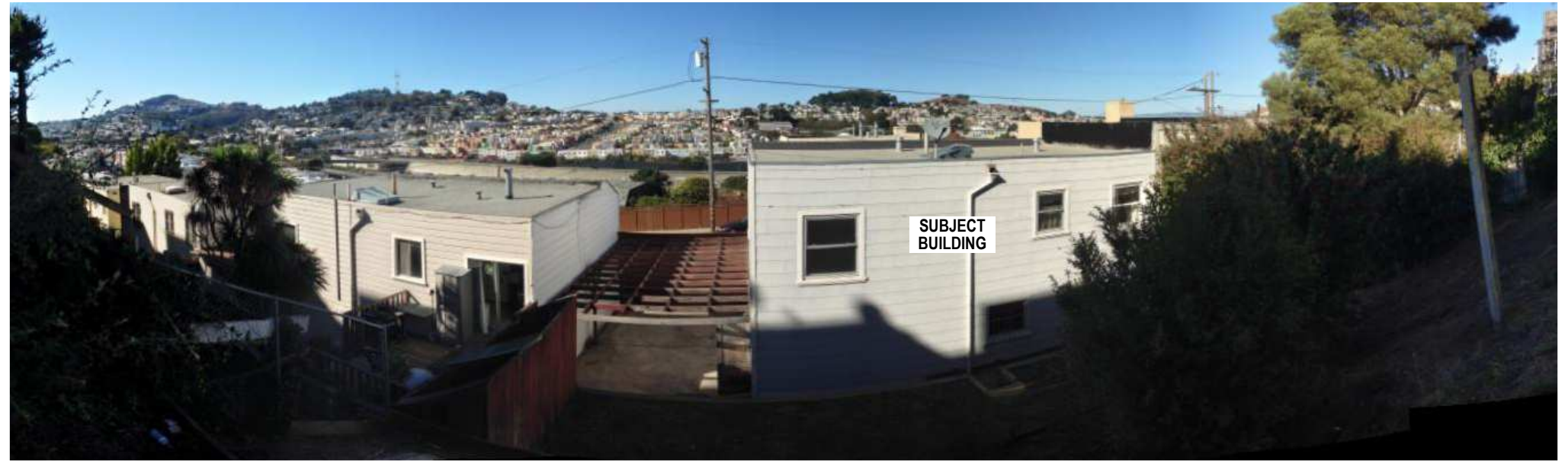
REAR FACADE OF SUBJECT AND ADJACENT BUILDINGS ALONG GLADSTONE DRIVE
