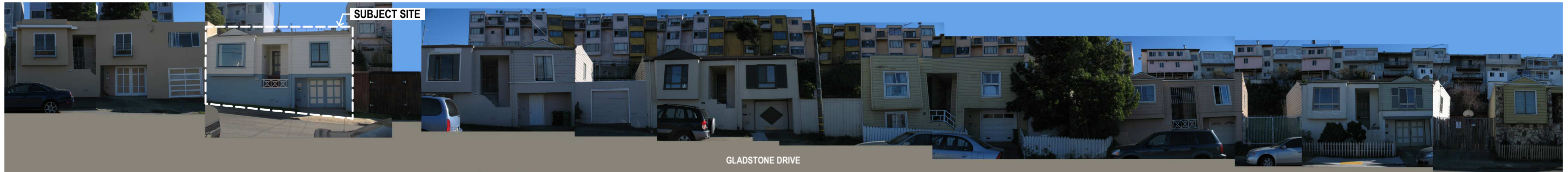
SUBJECT SITE AND ADJACENT BUILDINGS TO THE WEST ON GLADSTONE DRIVE (LOOKING SOUTH)
