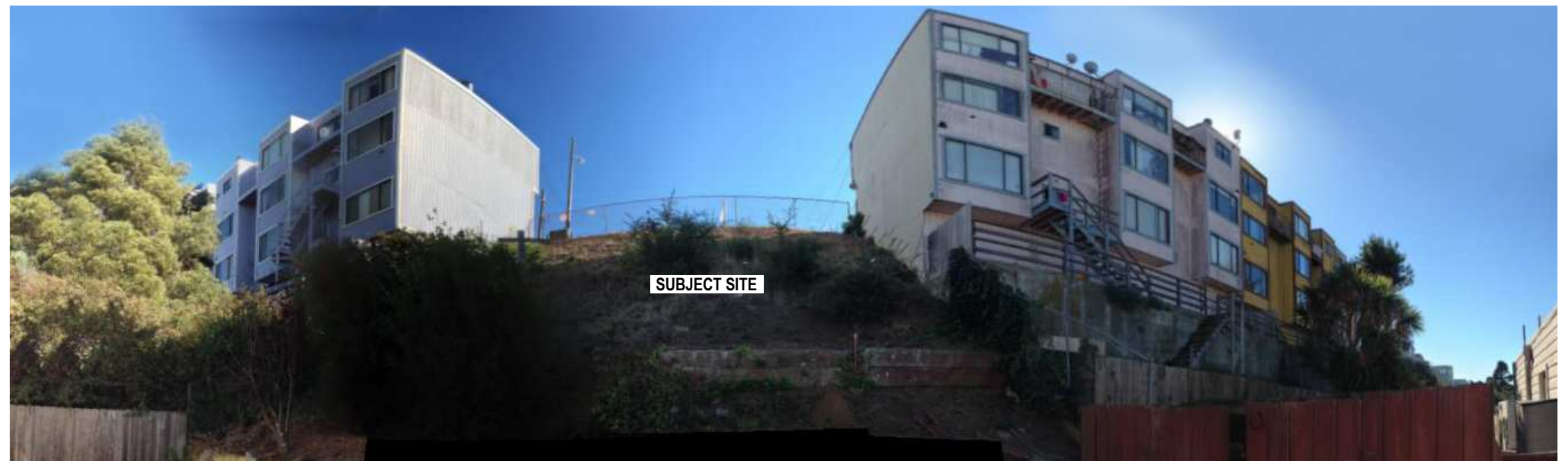
REAR FACADE OF ADJACENT BUILDINGS ALONG SILVER AVE
