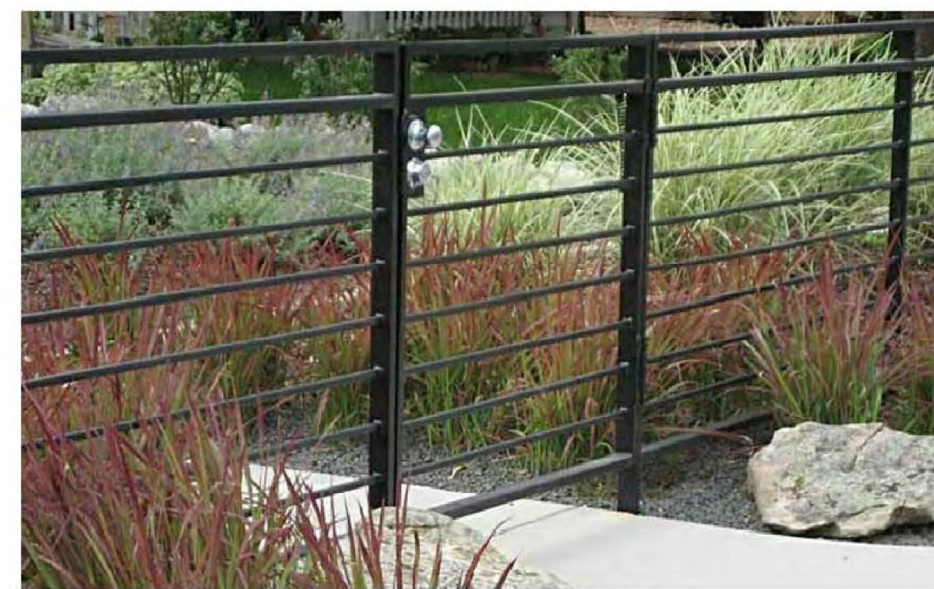
Ground Floor Private Terrace Fencing
