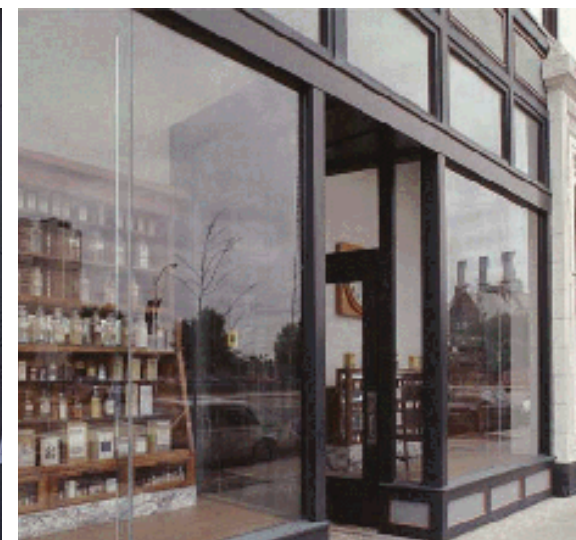
FLOOR TO CEILING WINDOW WALL 8
