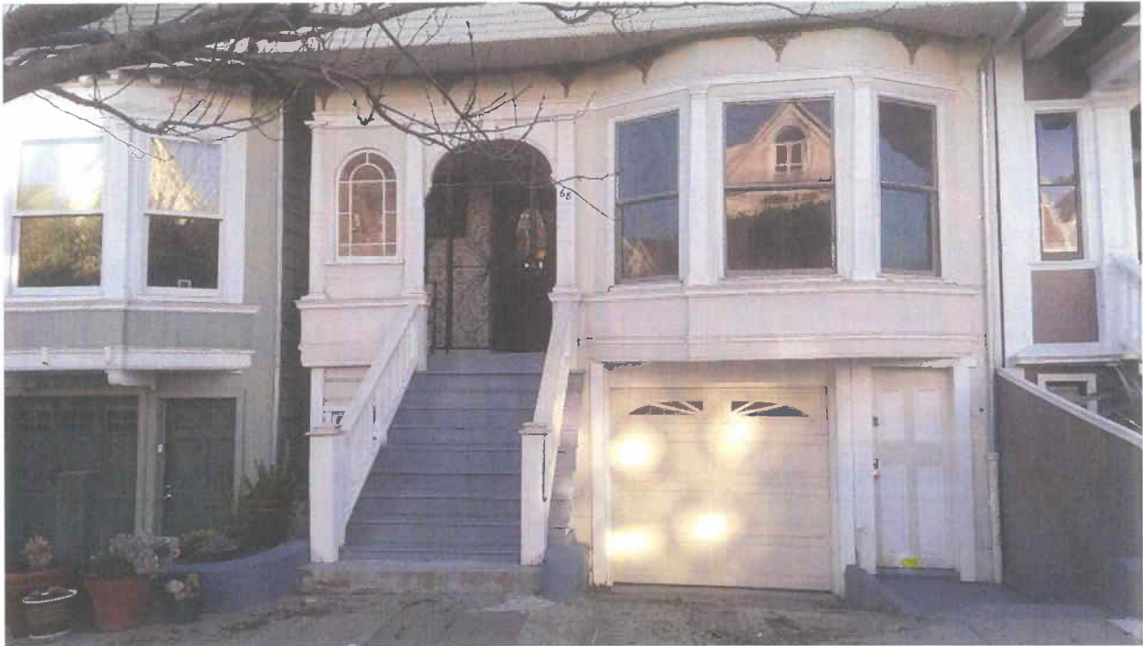
Lower part of front elevation
