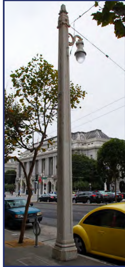
Van Ness trolley pole with single pendant
