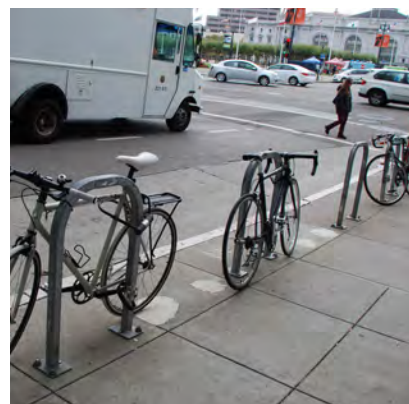
Bike rack - metal staple style, installed along Polk St
