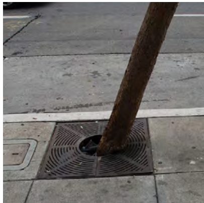
Square tree well with metal grate along Polk St
