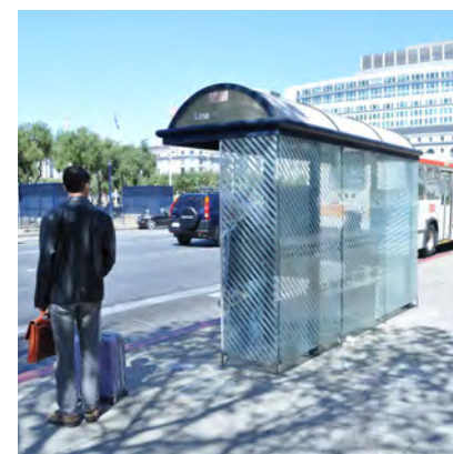
MUNI bus shelter with domed glass roof along Larkin St
