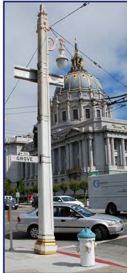
Van Ness trolley pole with single pendant and high pressure auxiliary water supply hydrant
