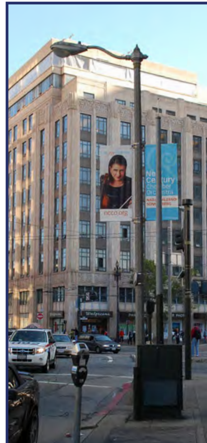
Aggregate concrete streetlight post with pendant arm style cobra luminaire at Larkin St
