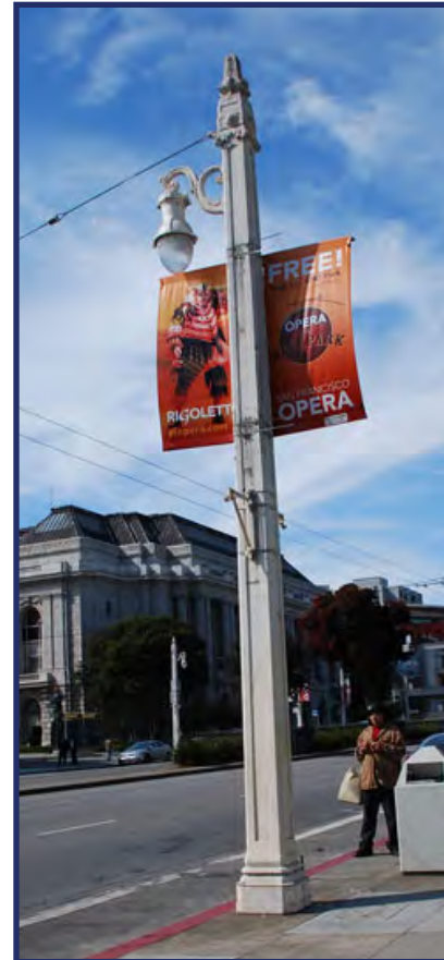
Van Ness trolley pole with single pendant
