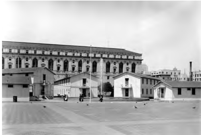
Figure 2.44 1943 image of paving detail of Civic Center Plaza with barracks and State Building in background (San Francisco History Center, San Francisco Public Library)
