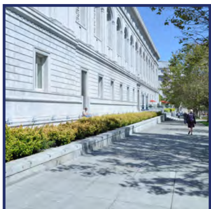
Planting area along Fulton Mall entrance
