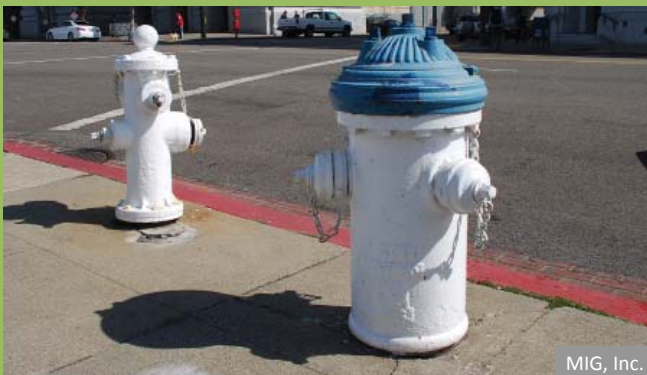
Auxiliary Water Supply System hydrant with a blue cap next to a low pressure hydrant near City Hall. Dates to 1909.
