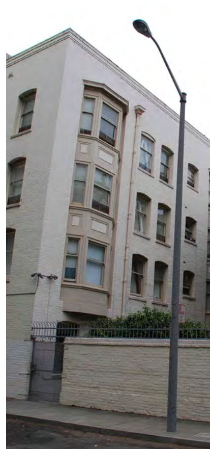
Single cobra street light on Redwood St
