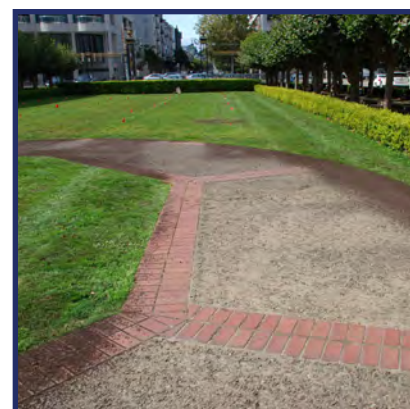
Detail of brick and aggregate path and lawn area at War Memorial Court
