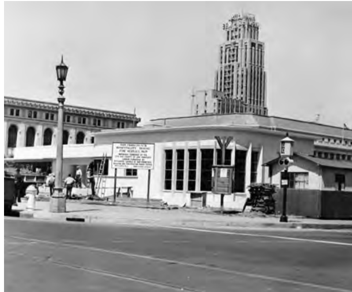
Figure 2.40 1941 Hospitality House construction with street lighting, fire hydrant and traffic signal (San Francisco History Center, San Francisco Public Library)
