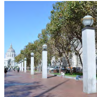
Square granite column lights with frosted globes along Fulton Mall
