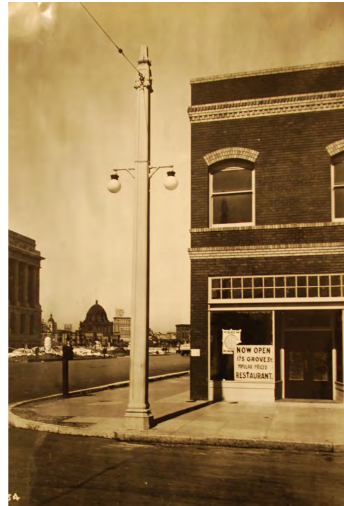
Figure 2.13 1915 Trolley Pole with lights (SF Dept. of Public Works historic photos, San Francisco History Center, San Francisco Public Library)
