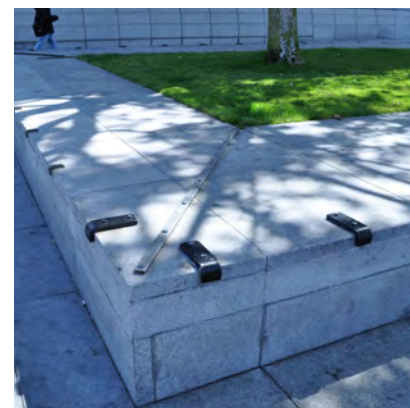
Elevated planting area and seat wall with skateboard deterrent clips at Larkin St
