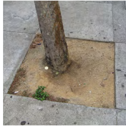
Square tree well filled with decomposed granite at Grove St
