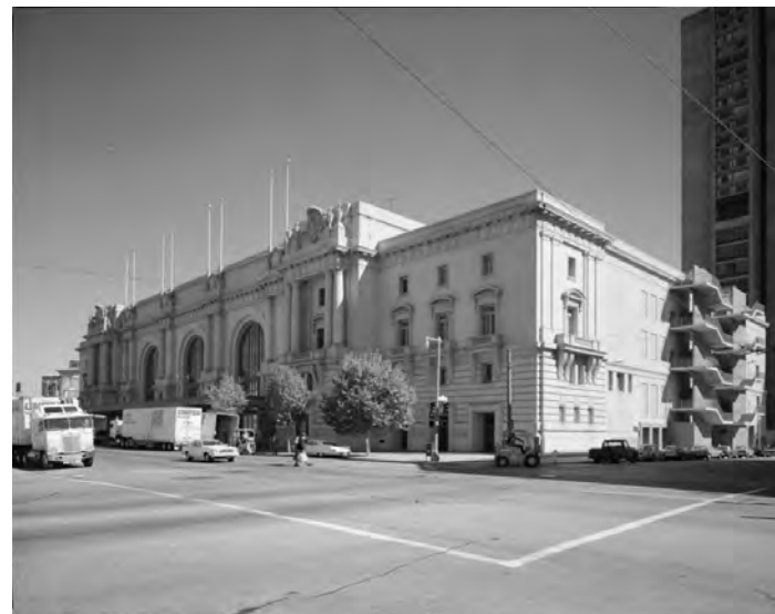
Figure 2.81 1981 Historic American Building Survey photo of Civic Auditorium at Grove and Polk Streets
