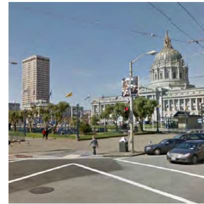
Overview of Civic Center Plaza from corner of Larkin and McAllister Streets*
