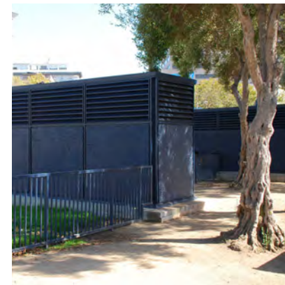
Brooks Hall ventilation structures near south playground along Larkin St
