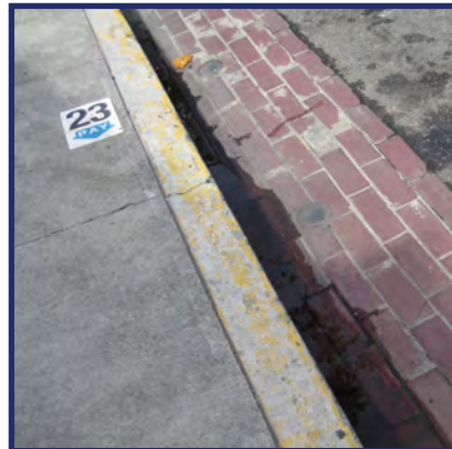
Granite curb with brick gutter along Grove St
