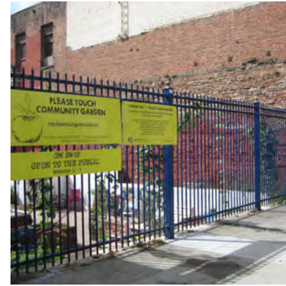
Blue painted metal fence along Grove St
