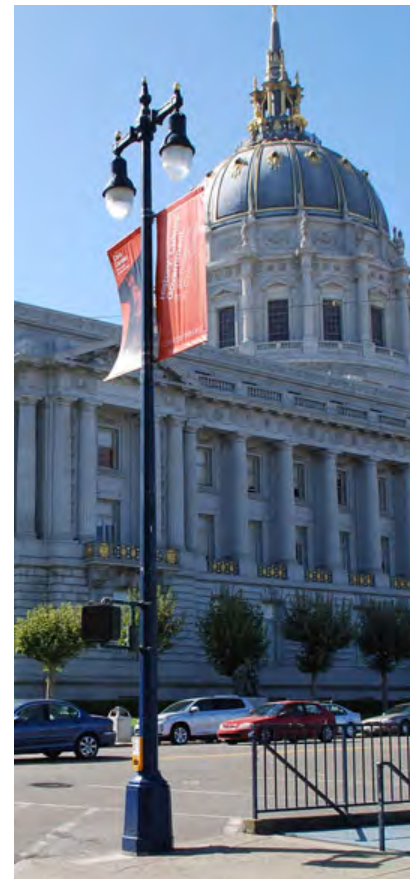
Street light - double pendant painted blue along Dr. Carlton B. Goodlett Place
