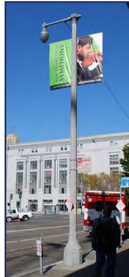
Aggregate concrete streetlight post with right angle pendant along Grove St
