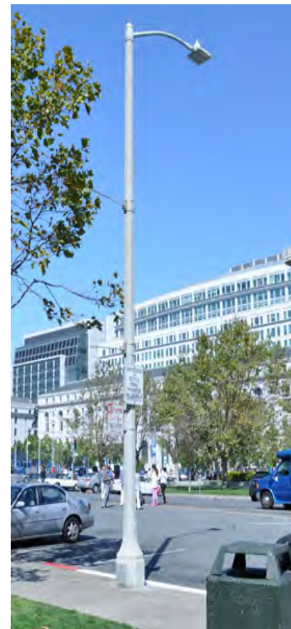
Single cobra street light along Fulton Mall
