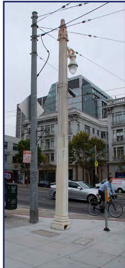
Van Ness trolley pole with single pendant
