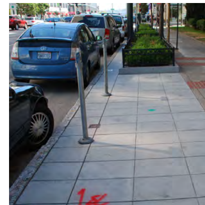
Concrete sidewalk with granite curbs along Van Ness Ave
