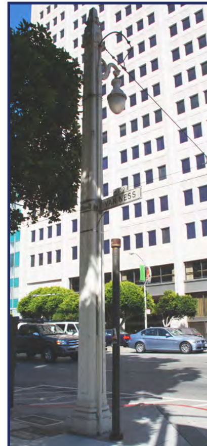
Van Ness trolley pole with single pendant
