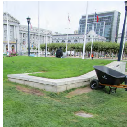
Retaining wall for display planting bed north of Exposition (Civic) Auditorium along Grove St
