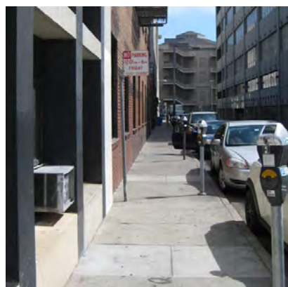
Concrete sidewalk at Lech Walesa St
