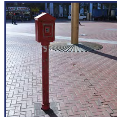
Fire box at UN Plaza and base of gold flag pole
