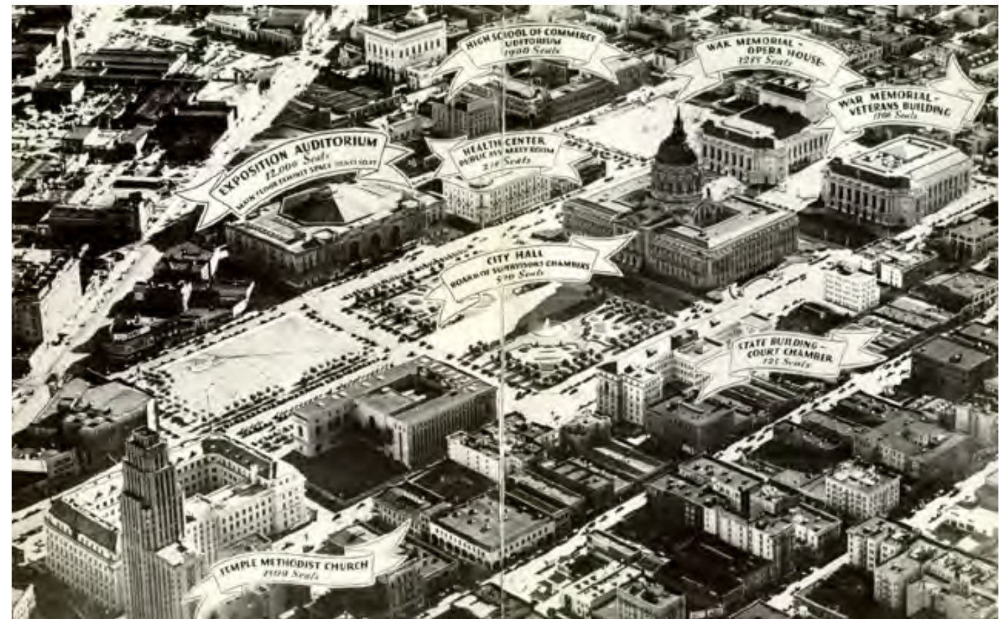
Figure 2.36 1930s annotated oblique aerial of the Civic Center district (San Francisco History Center, San Francisco Public Library)
