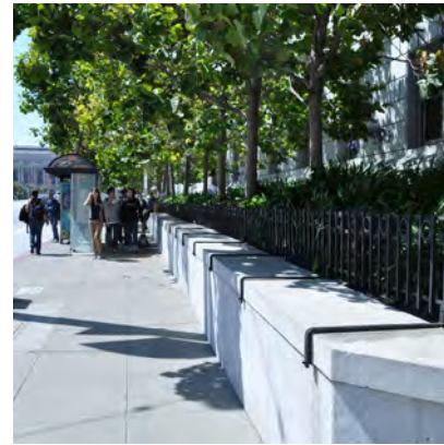
Elevated granite planter with anchored metal skateboard guards at Larkin & McAllister Streets
