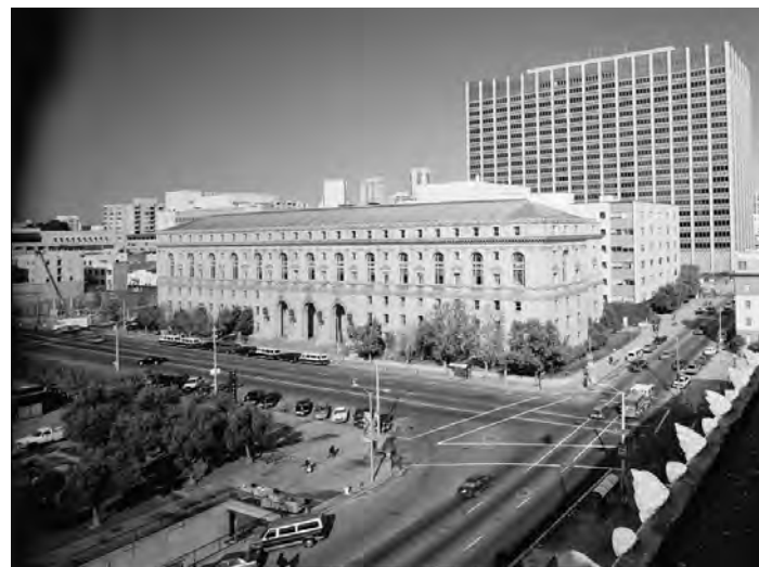
Figure 2.85 1995 Historic American Building Survey photo of State Building from the Public Library showing corner of Larkin Street and McAllister Street and NE corner of Civic Center Plaza
