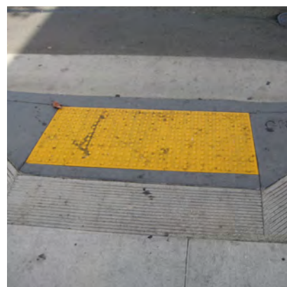
Accessible ramp with truncated domes
