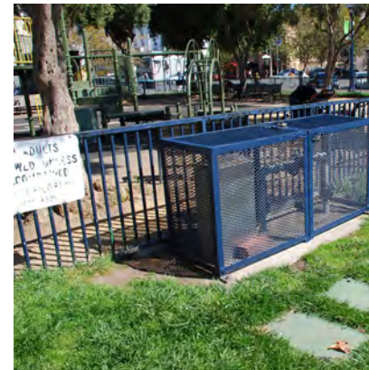
Blue painted metal utility cage near south playground
