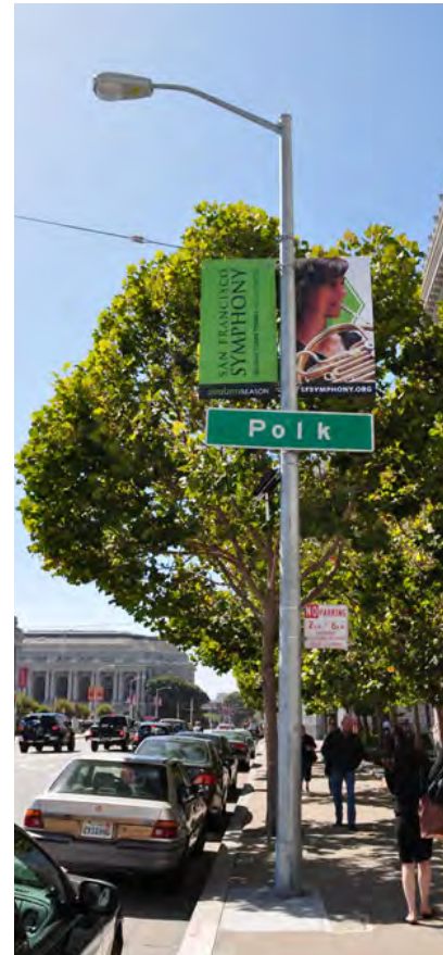
Single cobra street light with banners along McAllister St
