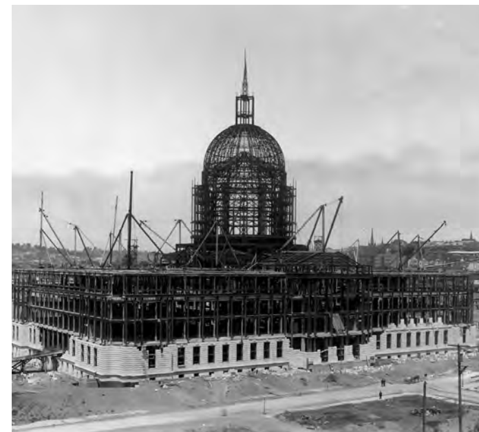
Figure 2.14 c. 1915 image of City Hall under construction (J. Tilman)
