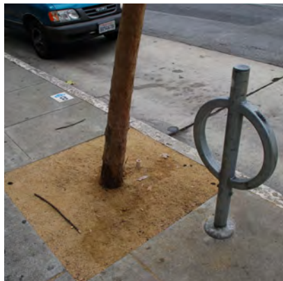
Square tree well with DG fill and ring and post style bike rack along Van Ness Ave
