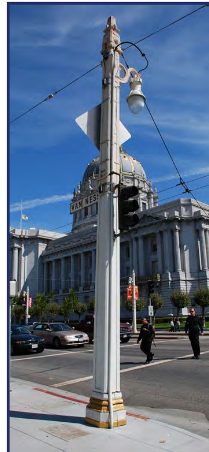
Van Ness trolley pole with single pendant
