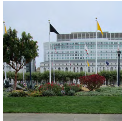
Elevated display planting bed and small flag poles north of Exposition (Civic) Auditorium
