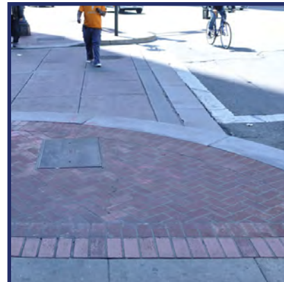
Granite curbs at Hayes St
