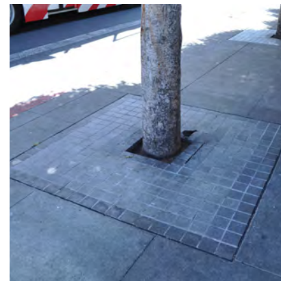
Square tree well filled with square tiles along Grove St
