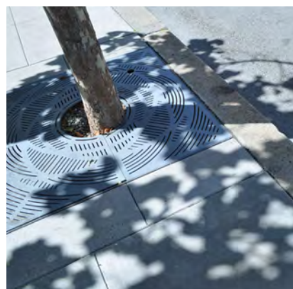
Square metal tree grate along McAllister St
