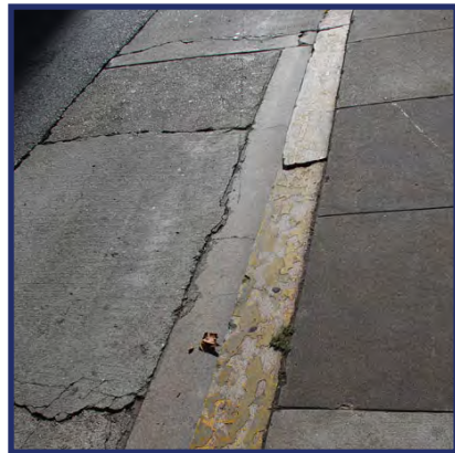
Granite curbs at Exposition (Civic) Auditorium block along Hayes St
