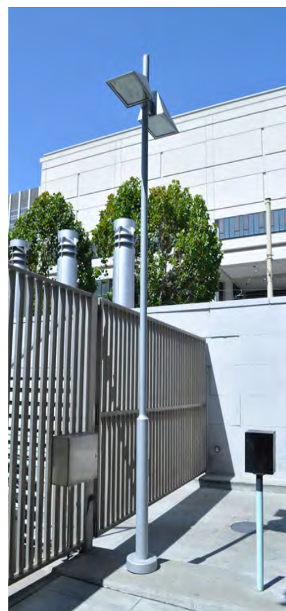
Light pole at Hyde St driveway and gate
