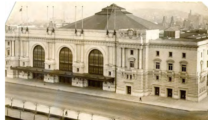
Figures 2.29 1924 photo of the Civic Auditorium (San Francisco History Center, San Francisco Public Library)
