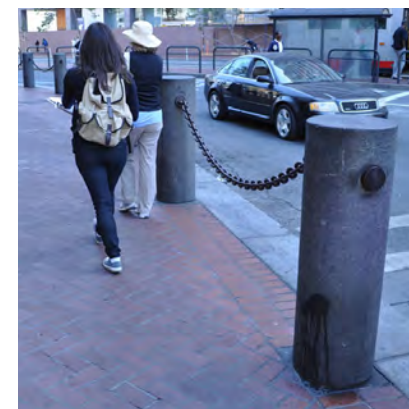
Granite bollards with chain along Hayes and Market Streets
