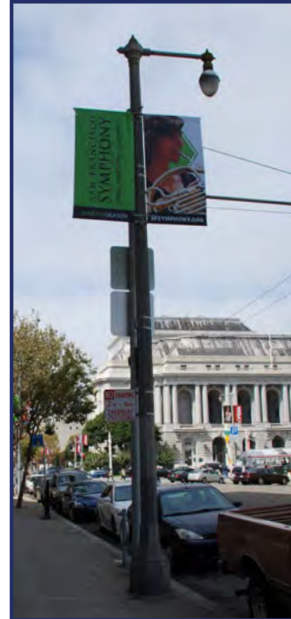
Aggregate concrete streetlight post with right angle pendant at Grove St
