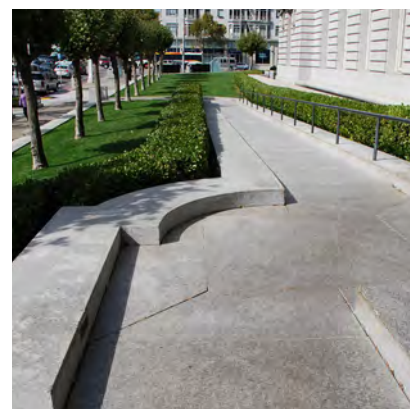
Accessible granite ramp to City Hall's west entrance at Van Ness Ave
