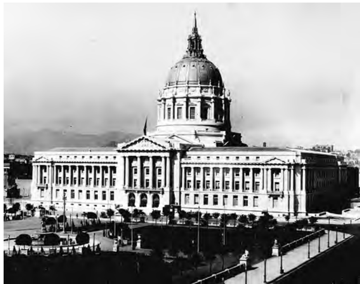
Figure 2.18 1915 image of City Hall with Civic Center Plaza in the foreground (J. Tilman)
