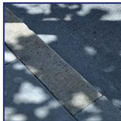
Granite curb along McAllister St
