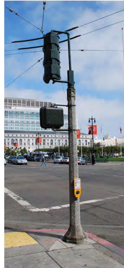
Modified aggregate concrete post with traffic signal
