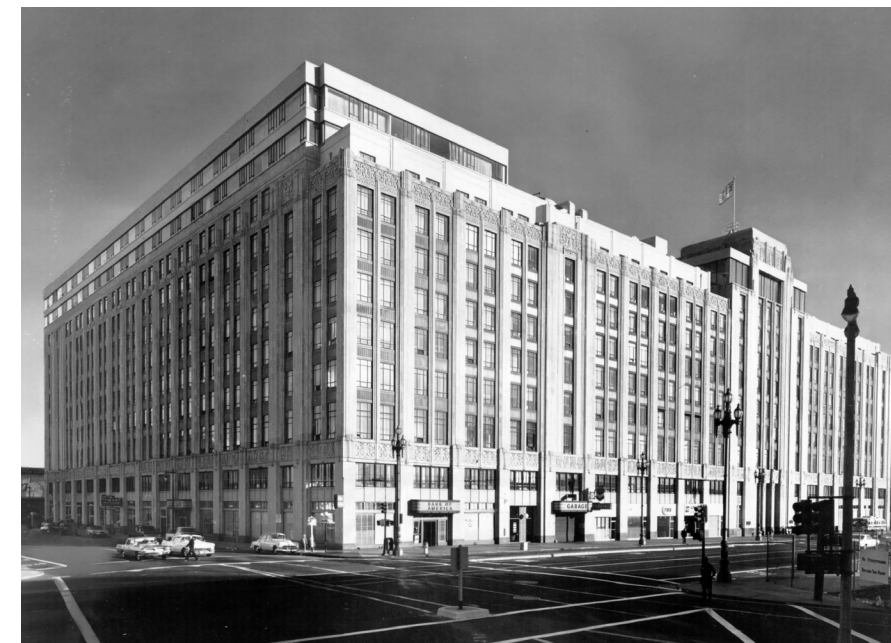
View southwest from corner of Ninth and Market Streets, 1965 [Note eleventh floor addition (1963)] (SFPL, #AAC-5017)
