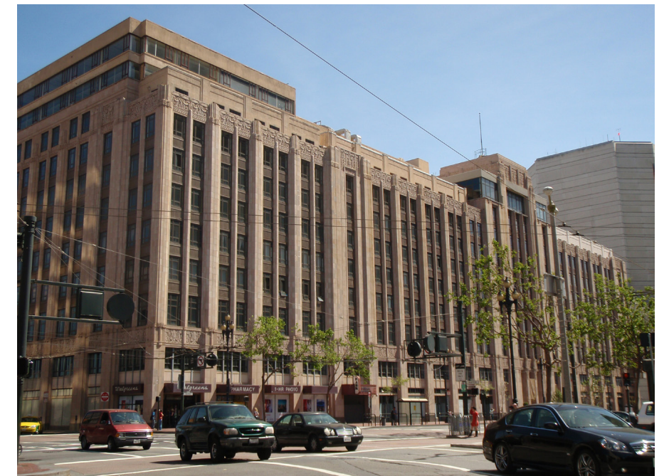
View of Market Street facade from Ninth Street, 2011
