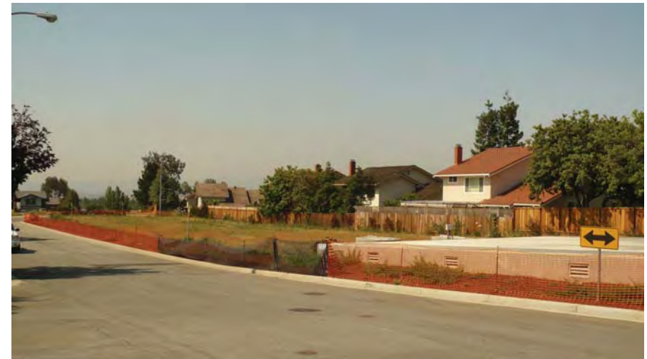
3d. SFPUC ROW and North Shutoff Station from Nugget Place and Tissiac Place looking southwest.
