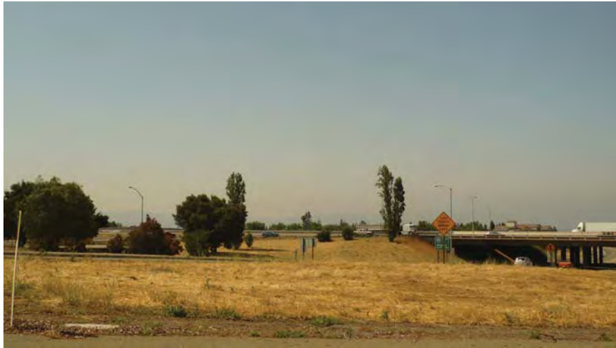
3a. Slip-joint vault and staging areas 2 and 3 from the Mission Boulevard/northbound onramp looking south.
