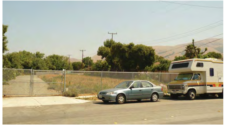
2b. South Shutoff Station from Crawford Street looking northeast.
