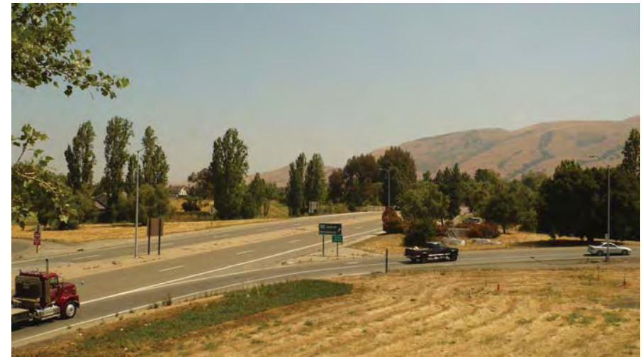
2d. Slip-joint vault and staging areas 2 and 3 from northbound I-680 looking north.
