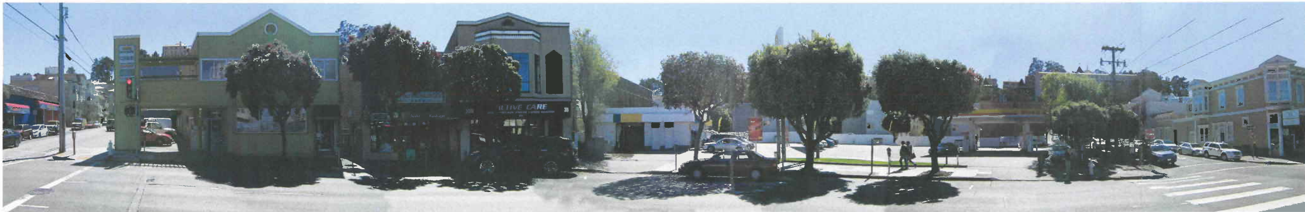
GEARY BLVD BETWEEN COOK ST AND BLAKE ST - FACING SOUTH
