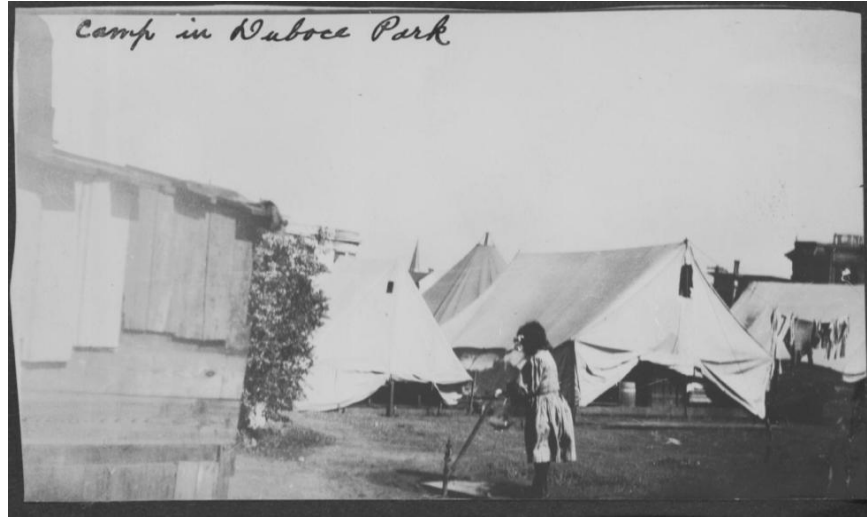
1906 Earthquake Refugee camp in Duboce Park. Source: California Historical Society.
