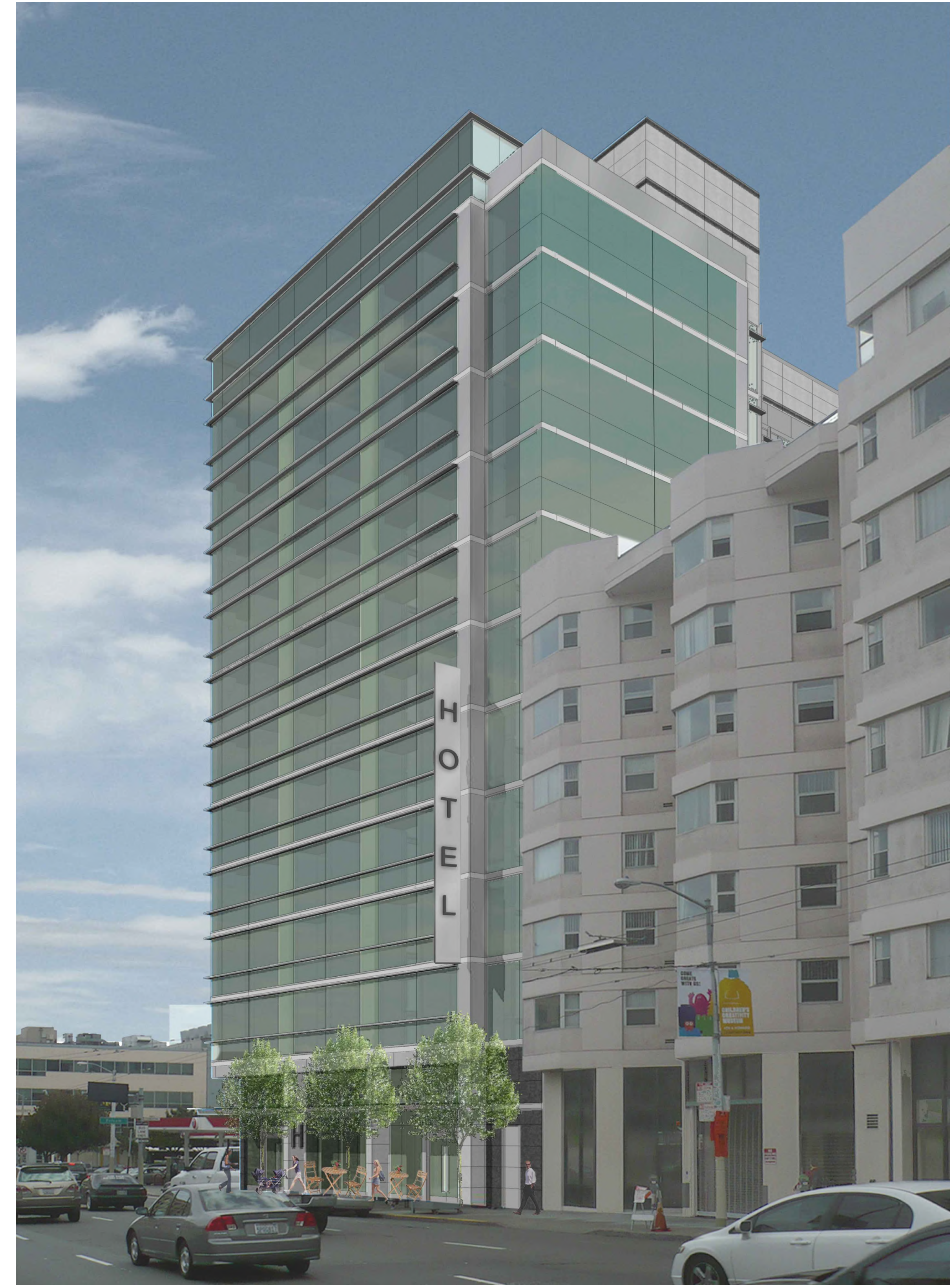
VIEW OF FOURTH STREET FACING SOUTH
