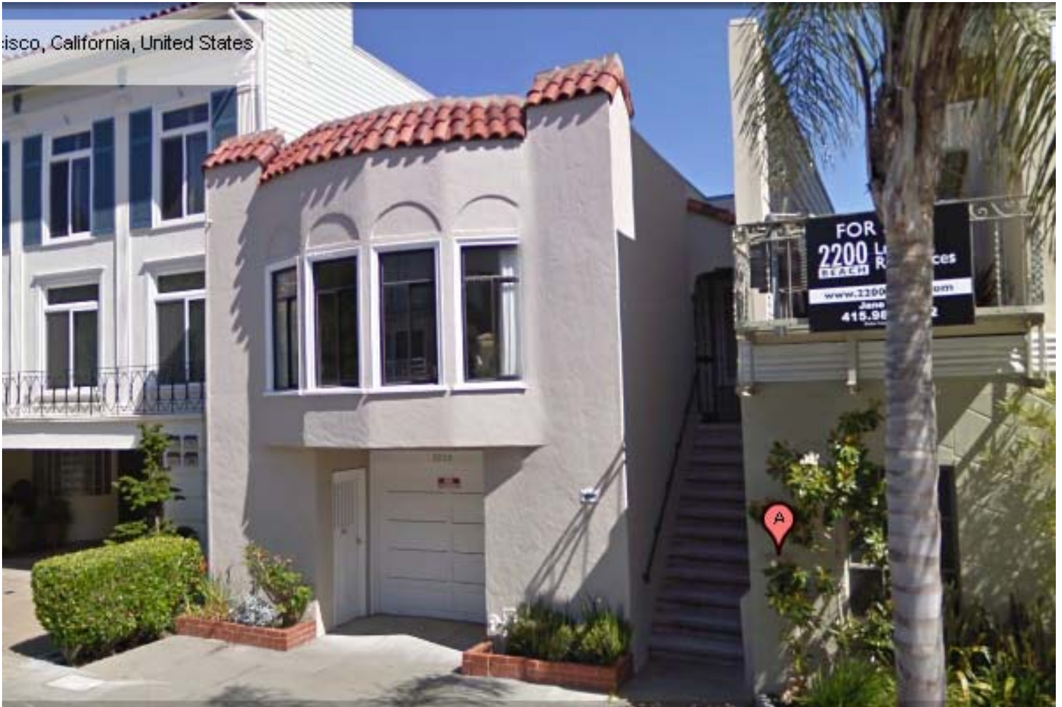
View of front facade looking northeast.
