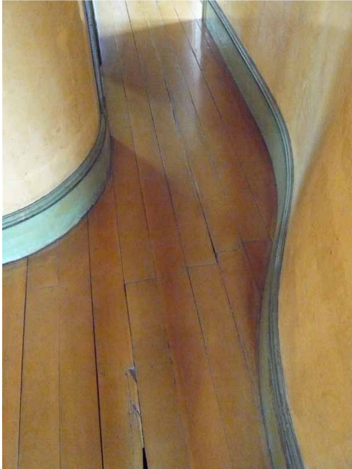
Detail of second floor hall
