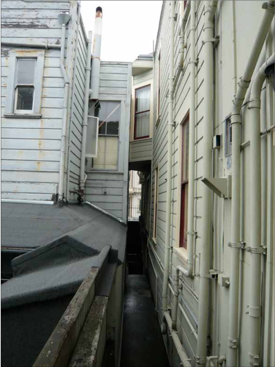
Detail of space between 500 Capp & 502-506 Capp Street
