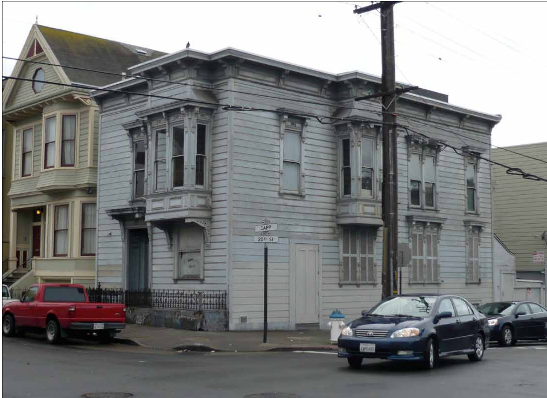
View from corner of Capp Street & 20th Street
