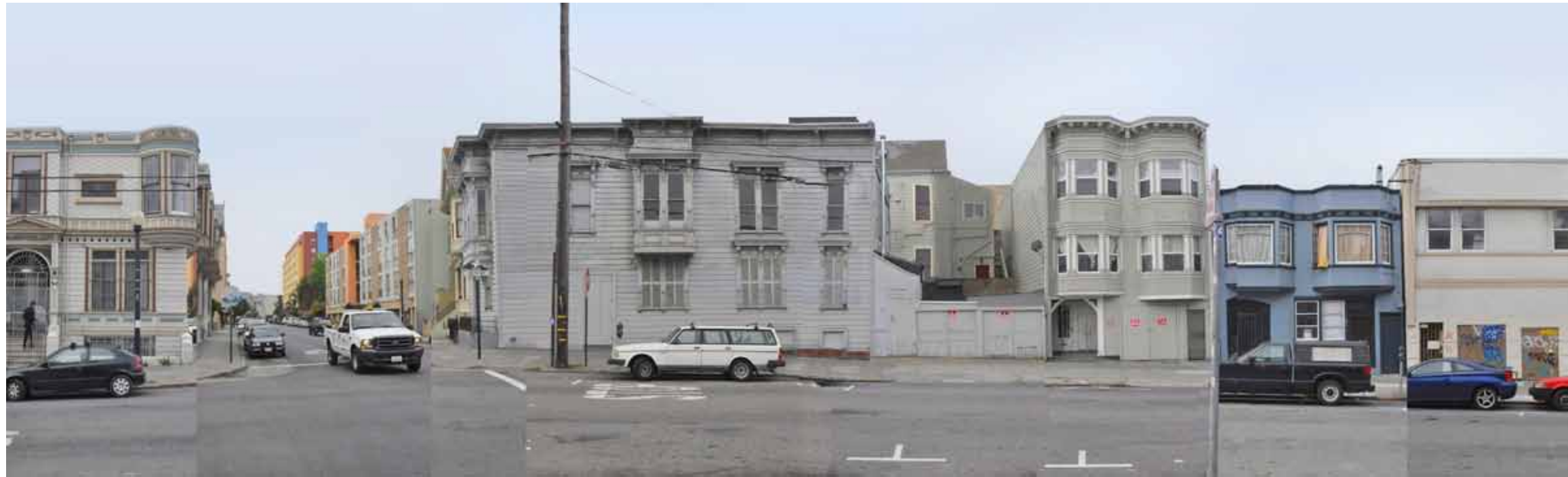
Existing 20th Steet Streetscape
