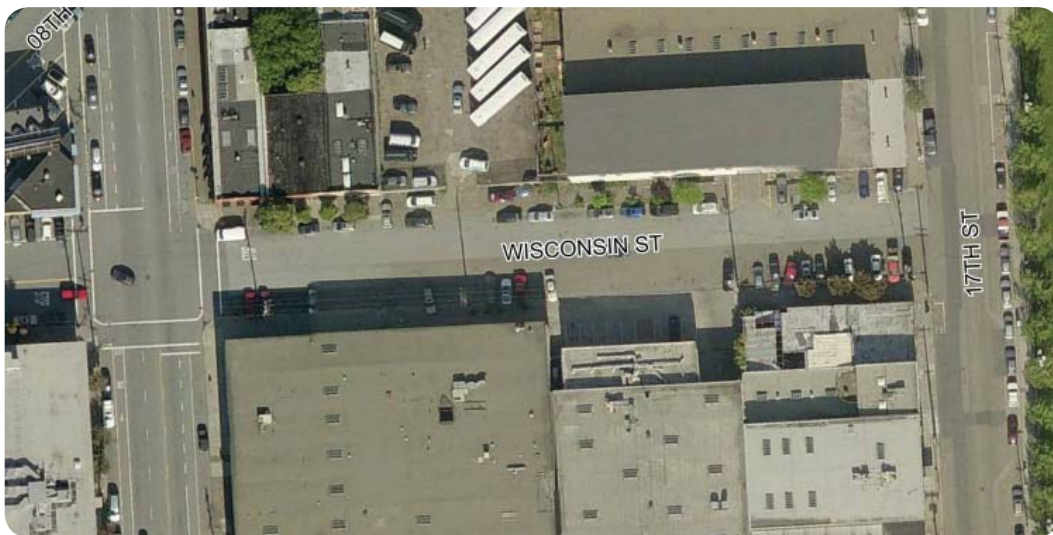
Figure C-11 Wisconsin Street – Existing Condition
