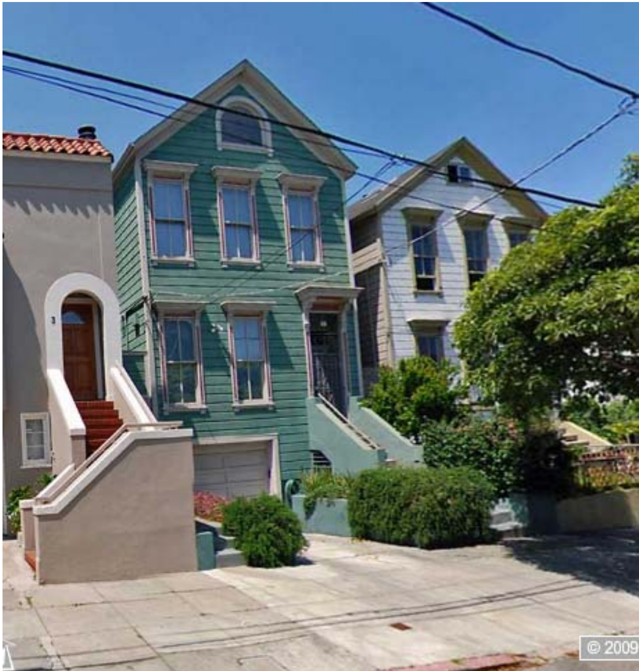
View of front facade looking northwest.
