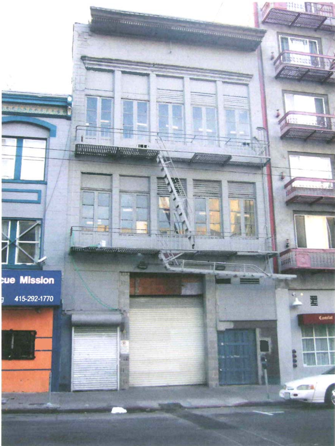
130 TURK STREET FACADE
