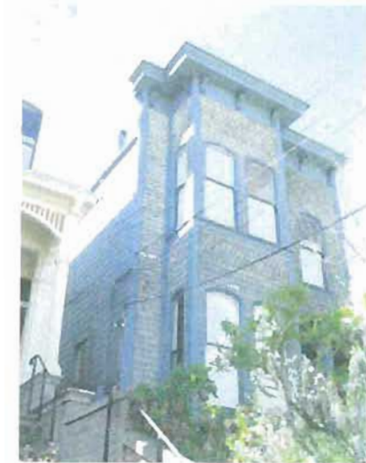
Oblique view of primary and secondary facades. Source: Page and Turnbull
