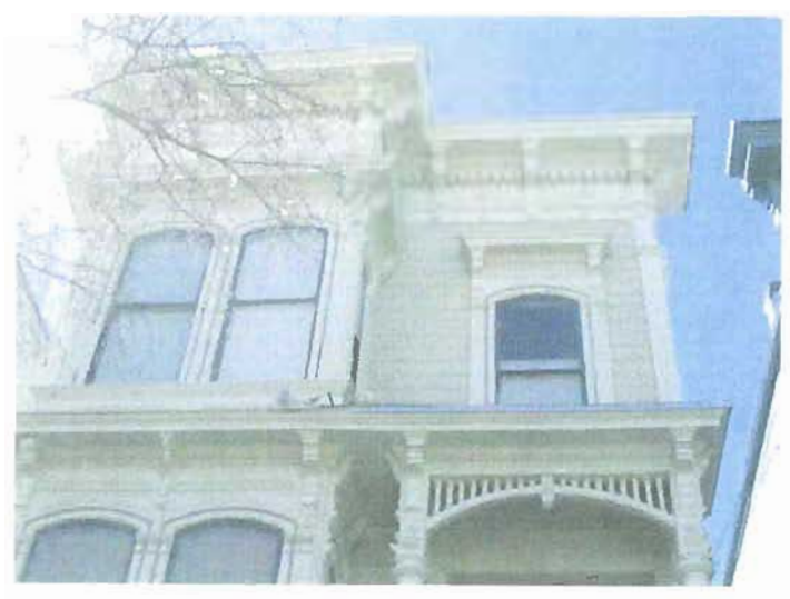
Detail of cornice. Source: Page and Turnbull
