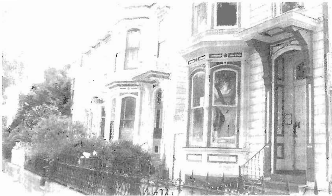
West side of Folsom Street south of 25 th Street.
