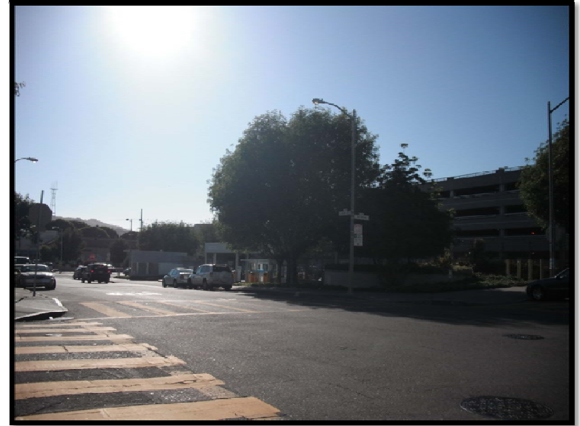
Figure 3 - Facing South Facade of Project Site from San Bruno & 24th Street
