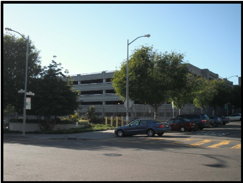
Figure 2 Facing South and East Facade of Project Site from San Bruno & 24th Street
