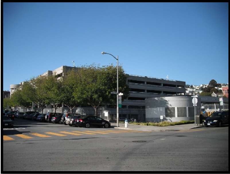
Figure 1 - Facing South & West facades of Project Site from Utah & 24th Street
