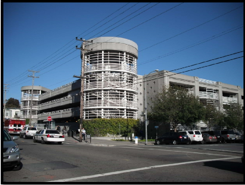
Figure 5 - Facing Northwest corner of project site from Utah & 23rd Street
