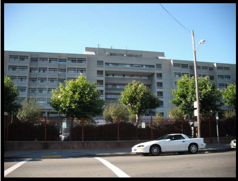
Figure 21 - Facing North from San Bruno & 23rd Street
