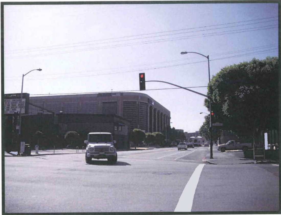
Figure 9 - Facing Southeast from Brannan/8th Street
