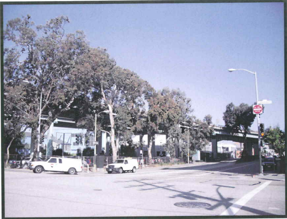
Figure 3 - Facing Northwest from Brannan/8th Street
