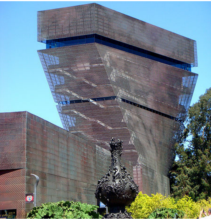
Across the concourse from the California Academy of Sciences, the De Young Museum presents less hazards due to its low amount of glazing and perforated copper facade.
