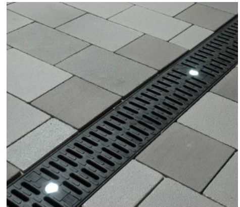
ABOVE: Grates on the ground should be smaller than 2 cm x 2 cm to prevent the trapping of stunned birds.
