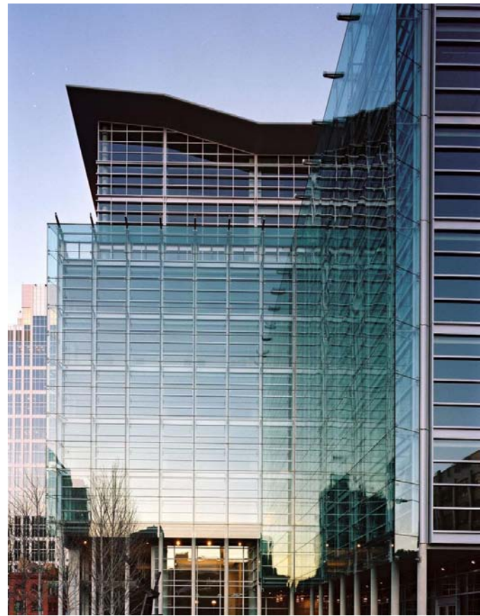
TOP: Foundry Square presents a full façade of highly reflective glass. While all glass can be reflective, glass manufacturers label glass with standards “reflectivity” ratings.
