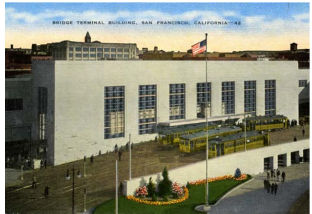
ABOVE: Many historic buildings such as the old Transbay Terminal present a solid appearance.
