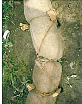
detail of wattle, rope, and wooden stakes
