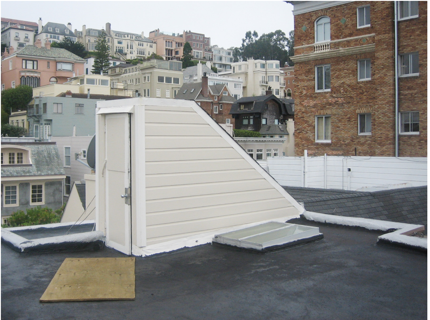
EXISTING STAIR PENTHOUSE OF 2768 GREEN STREET
