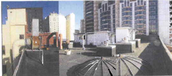
4 VIEW FROM SW CORNER LOOKING NE
