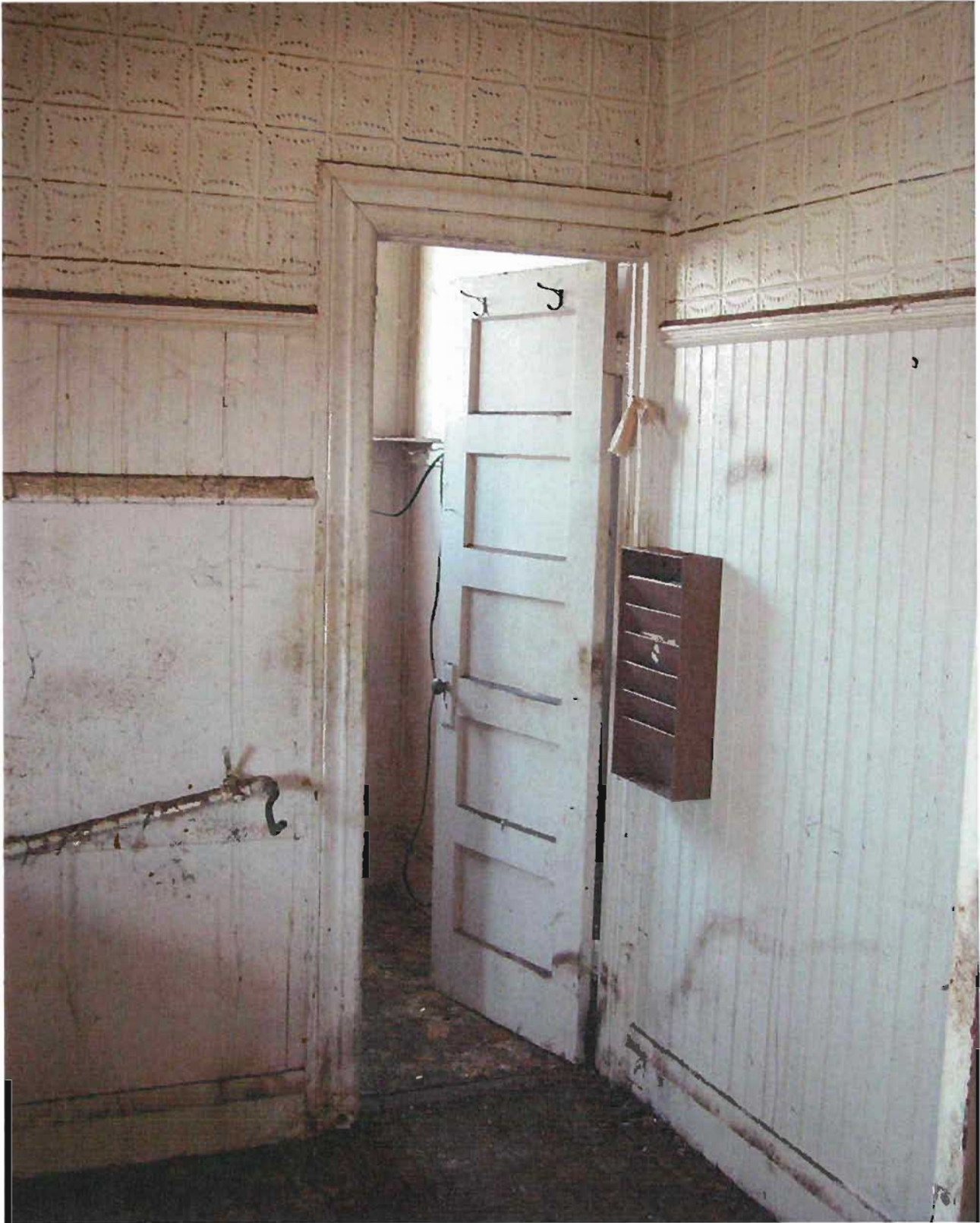
EXISTING BEL ROOM
