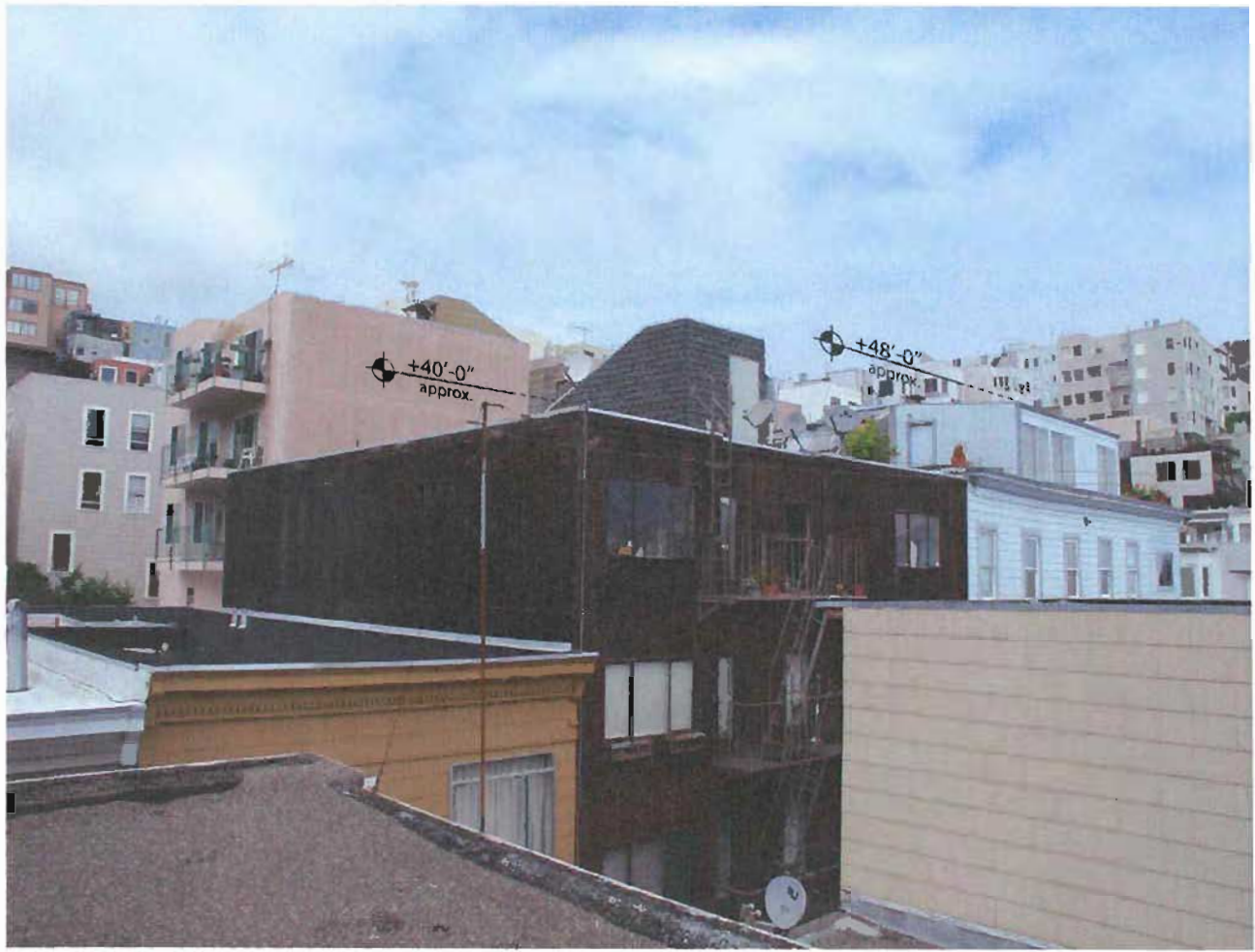
VIEW LOOKING NORTHWEST FROM 39 1/2 PRESSCOTT COURT
