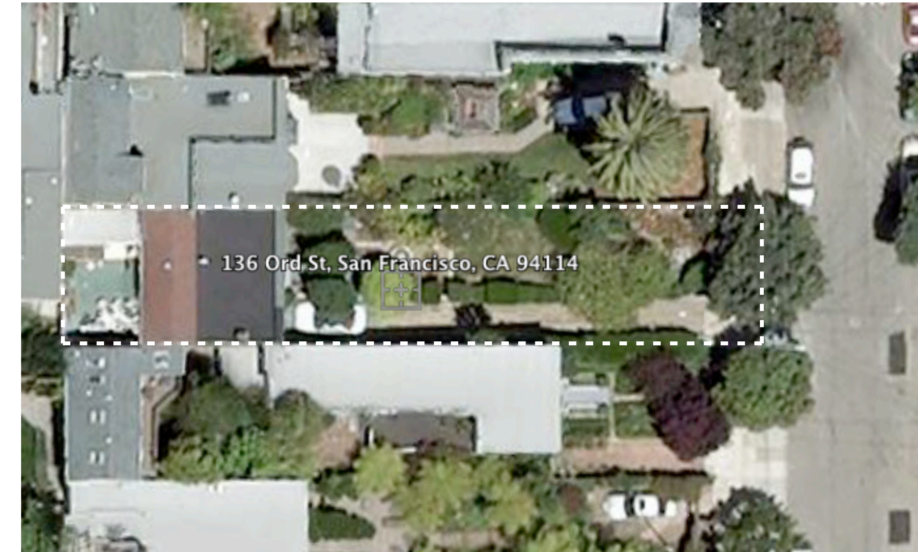
1 AERIAL PHOTO OF SUBJECT LOT
