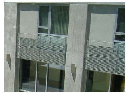
9 METAIL GUARDRAIL, PAINTED
