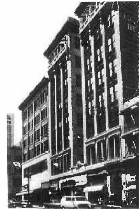
1000 HYDE STREET, SAN FRANCISCO, CALIF. ARCHITECT JOHN C. STETSON, 1910
