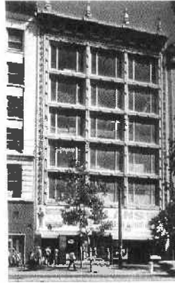
113-115 NORTH MARKET STREET, JOHNSON BUILDING, ARCHITECT W. W. R. B. 1911
