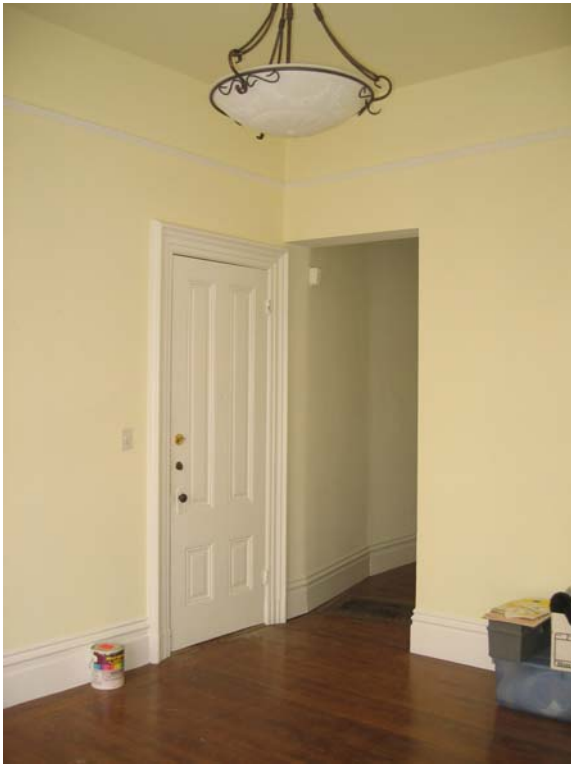
The vestibule wall cuts off the unit from the stair, further disengaging the two levels. The angled walls are an obvious afterthought.
