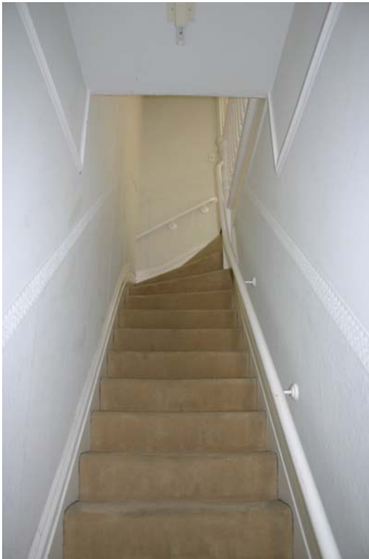
The steepness and narrowness of the stair is amplified by the solid wall. It could be opened up by removing the wall and the closet above.
