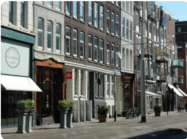
Outward facing buildings with good building elements
