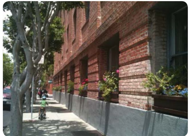
Articulated building with well-defined base
