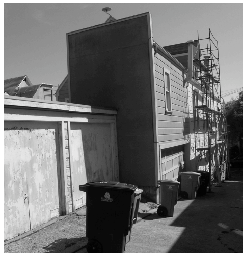
2 PHOTOGRAPH OF SITE
