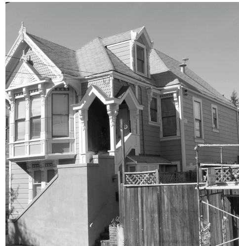
5 PHOTOGRAPH OF SITE
