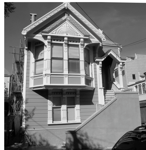
6 PHOTOGRAPH OF SITE
