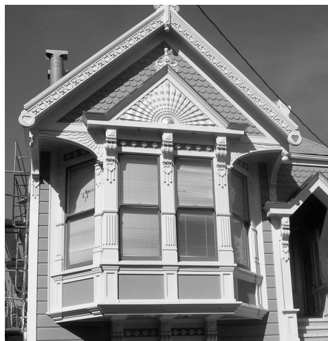
3 PHOTOGRAPH OF SITE
