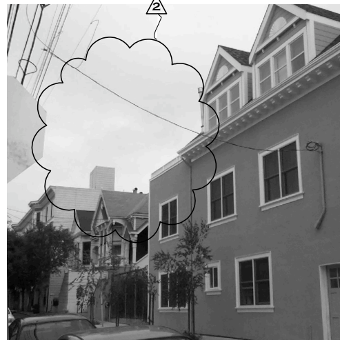
1 PHOTOGRAPH OF SITE
